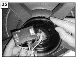
Loosen the 2 screws with key slots and remove the screw without key slot. Pass plug and capacitor through hole in plate. Take plate and place over the 2 screws with key slots and twist to hold in place.
